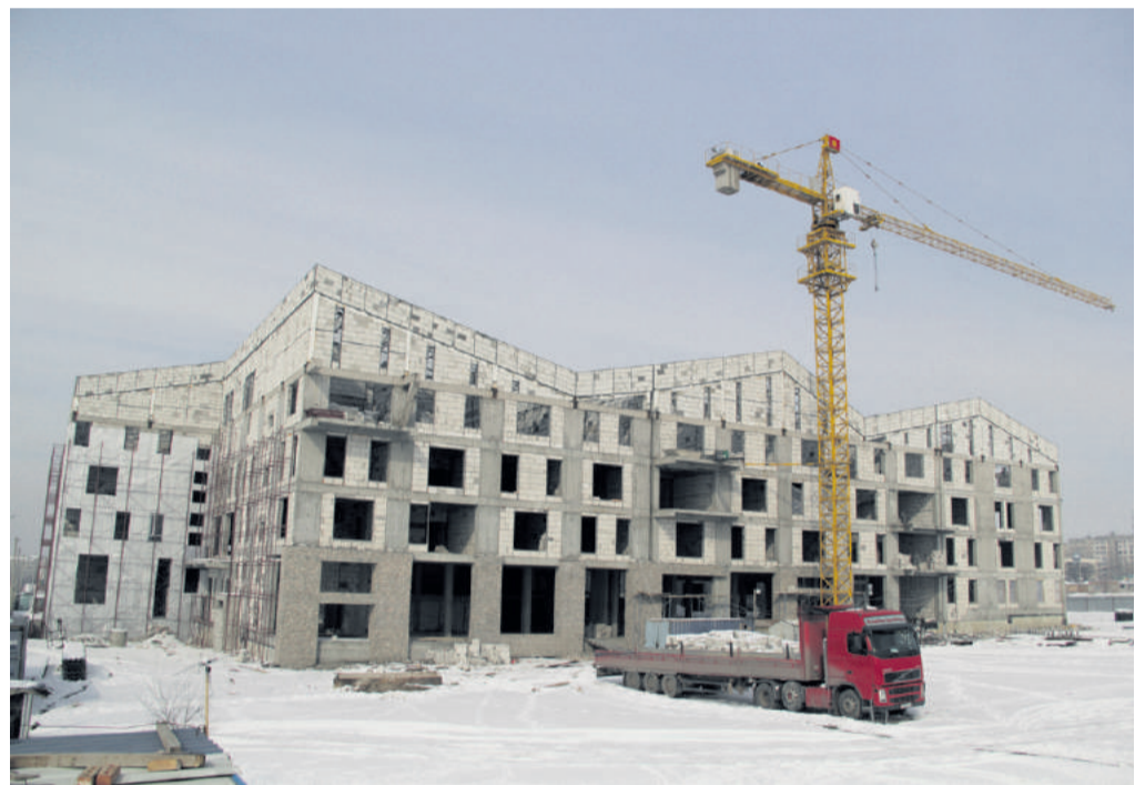
Campus construction process, February, 2014 Photo by Masha Panfilenko
